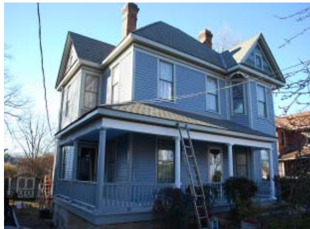
Restoring original wood siding allows the opportunity for new paint colors.
