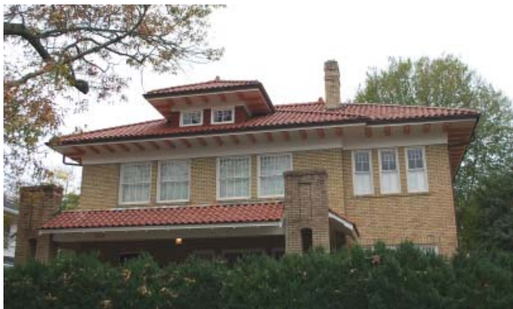
Terra cotta, tiles are a defining feature of this house in Fisher Park. A slate or clay tile roof can last 100 years or longer with routine maintenance.
