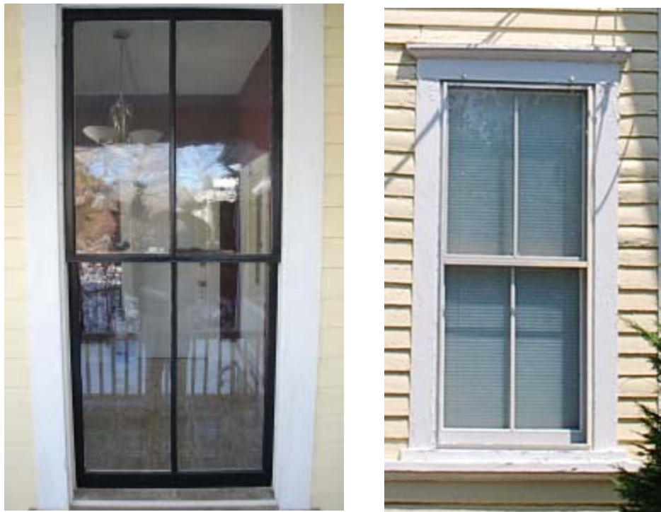
Original windows (left) have a character that is missing in replacement windows (right). This character is derived from the wavy hand made glass, wood joinery, and the operating components.
