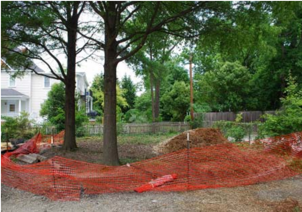
Trees should be protect trees during construction.
