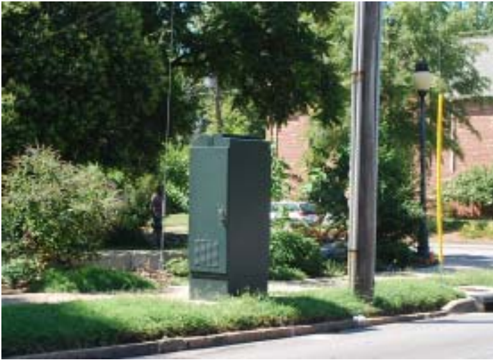
When new traffic signal control panels were planned, a dark green color was used for those in the historic districts to make them less noticeable.
