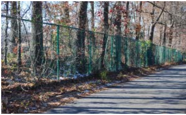
This vinyl coated chain link fence was installed along Oakland Avenue and the railroad tracks that border the neighborhood on the south in the College Hill Historic District.
