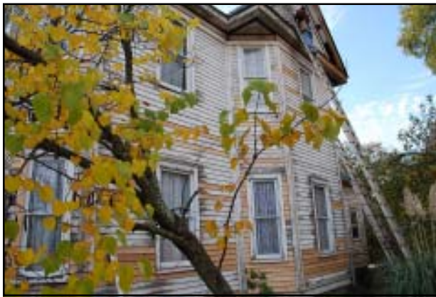
Wood siding that was damaged during installation of aluminum siding was replaced with new wood siding to match the original.
