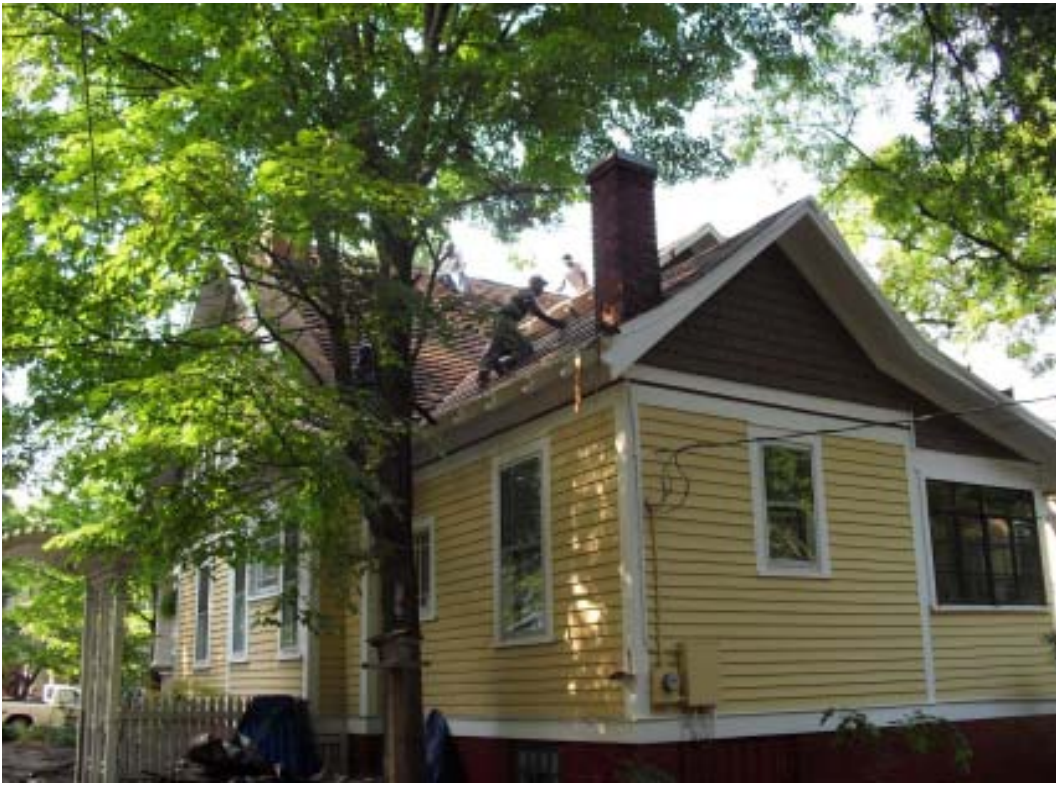
This house in the Aycock Historic District was roofed originally with wood shingles. Over time the wood shingles were covered with asphalt shingles . Both layers of shingles were removed revealing the nailer strips for the wood shingles. Plywood sheathing was installed over the nailer strips and new fiberglass shingles put down.
