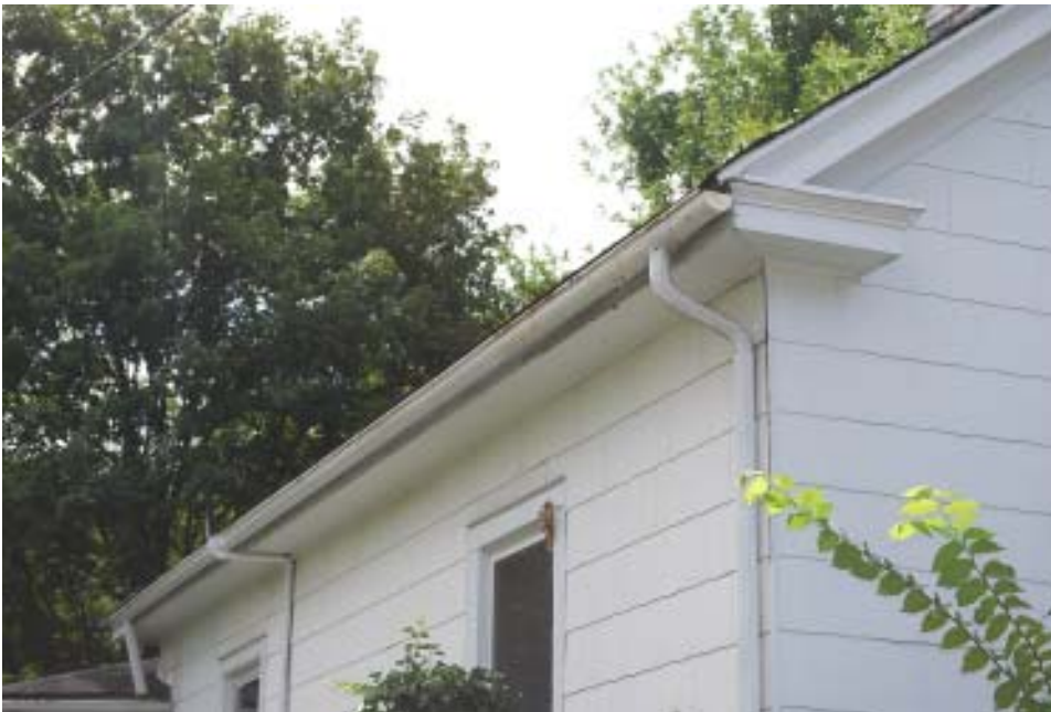
Half round gutters were used on buildings with decorative crown molding. Because they are fastened to the roof itself they do not require a flat surface like modern K-style gutters and do not require removal of crown molding.
