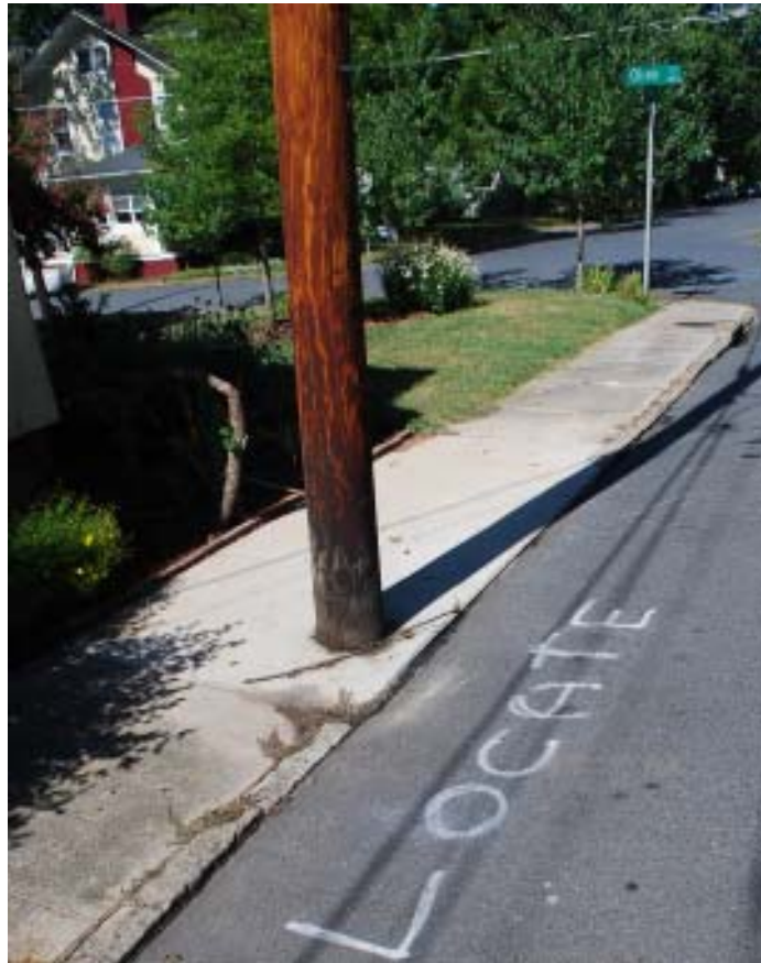
Too often the granite curbing is being lost through utility work such as replacement of poles or underground service lines.
