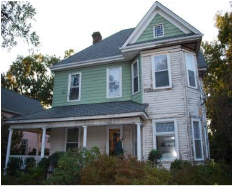
Removing substitute siding and repairing original wood siding and trim can restore the original character of an old house that was hidden for many years.
