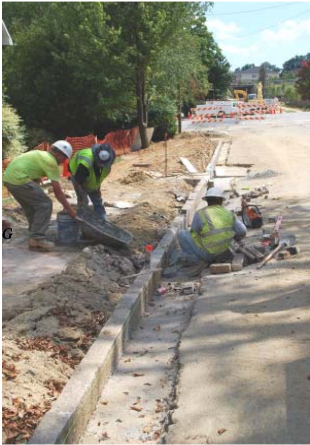
After they were taken up so that storm sewer pipes could be replaced in College Hill the granite curbing was re-set and the brick gutters re-laid.
