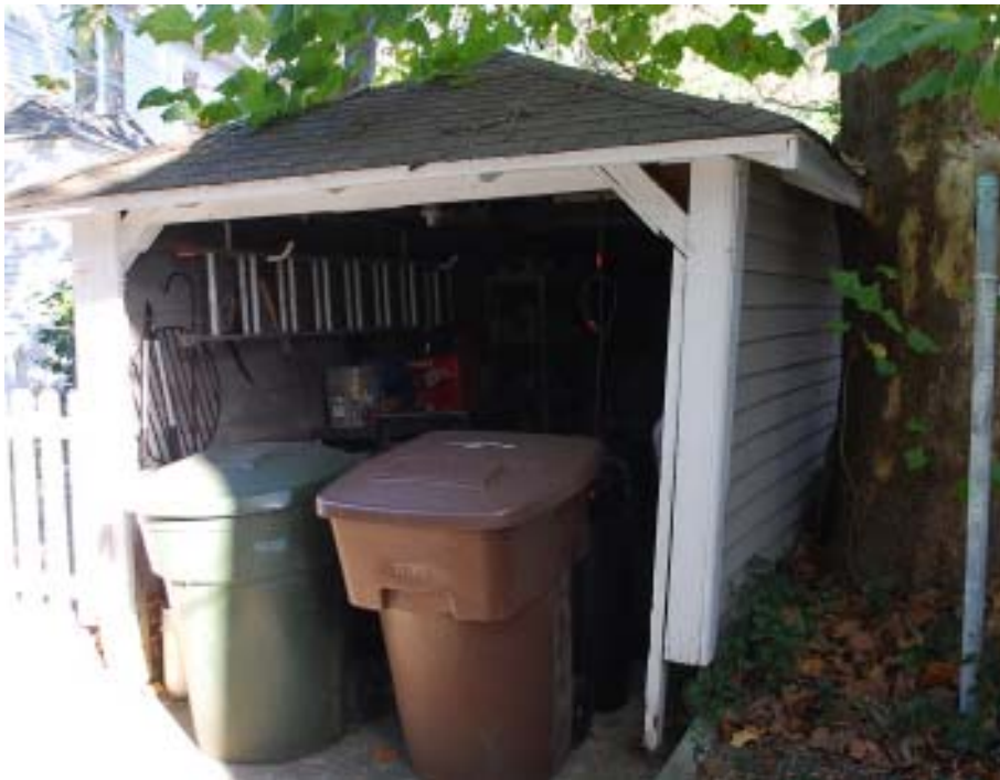
Early garages were designed for automobiles that were smaller than modern vehicles. They were usually not built on foundations so they were prone to deterioration.
