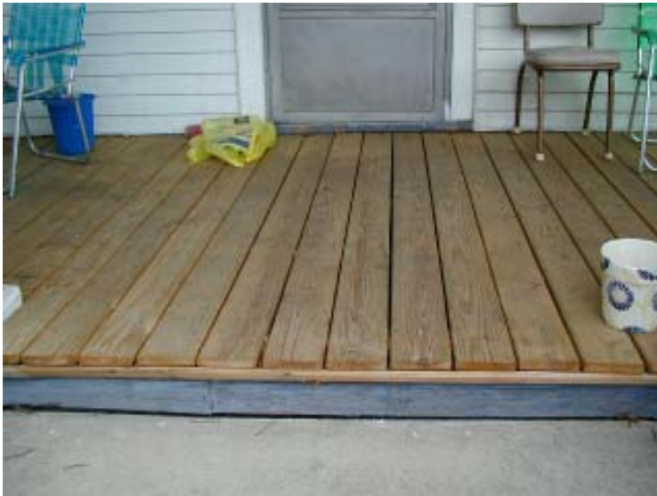
The original tongue-and-groove porch flooring was replaced with treated deck boards. Besides losing some of the historic character of the porch, water can now leak through the spaces between the boards and cause deterioration for structural framing.
